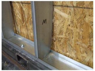
Missing fasteners at the bottom
