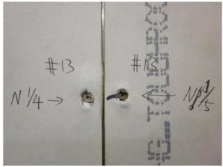
Vertical seam fasteners
